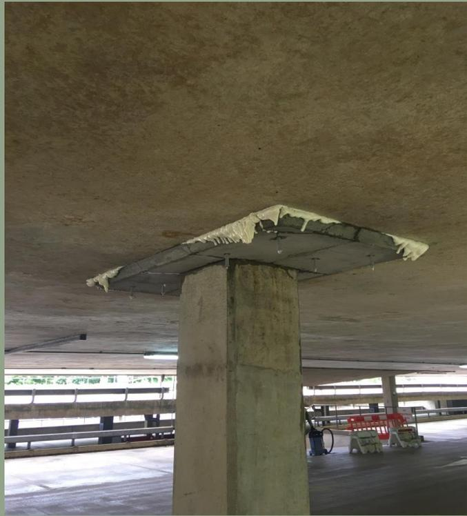
Delaminated column top thickening overhead requiring *Structural Resin Bonding* using our pressure injection system. Preventing the concrete thickening from spalling and to seal the head from water ingress through the top deck column lift slab.
